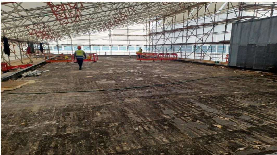
Images above: progress on Town Centre House
