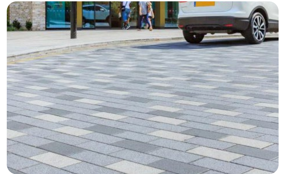
(03) Vehicle crossovers, mixed colour stone aggregate concrete flags. Ensure deep construction to allow for vehicle overrun.
