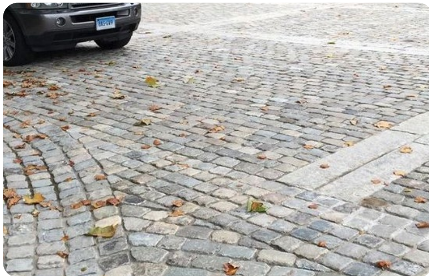
(04) Carparking pavement with small granite cobblestones, ensure deep construction to allow for vehicle overrun.
