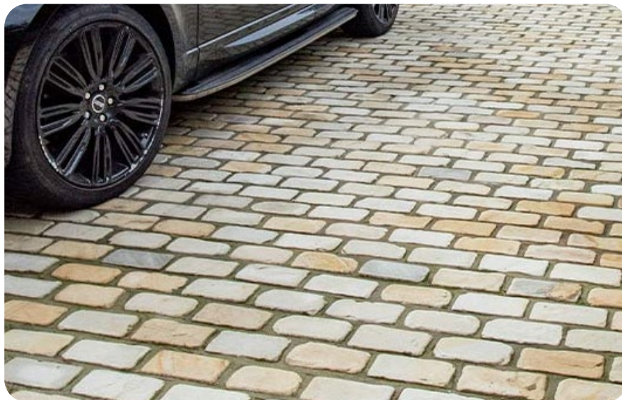
(04) Carparking pavement with small yorkstone blocks, ensure deep construction to allow for vehicle overrun.
