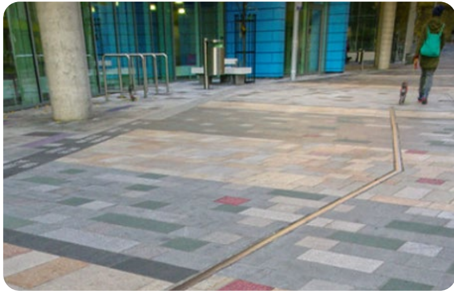
(01) Improved paved footways using manmade stone aggregate concrete flag pavers.
