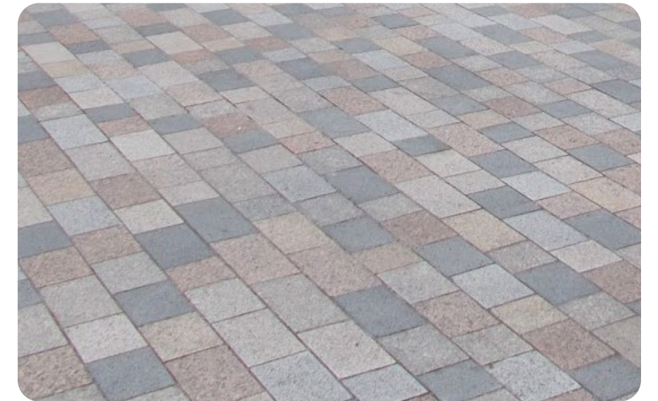
(03) Vehicle crossovers, mixed colour granite pavers. Ensure deep construction to allow for vehicle overrun.
