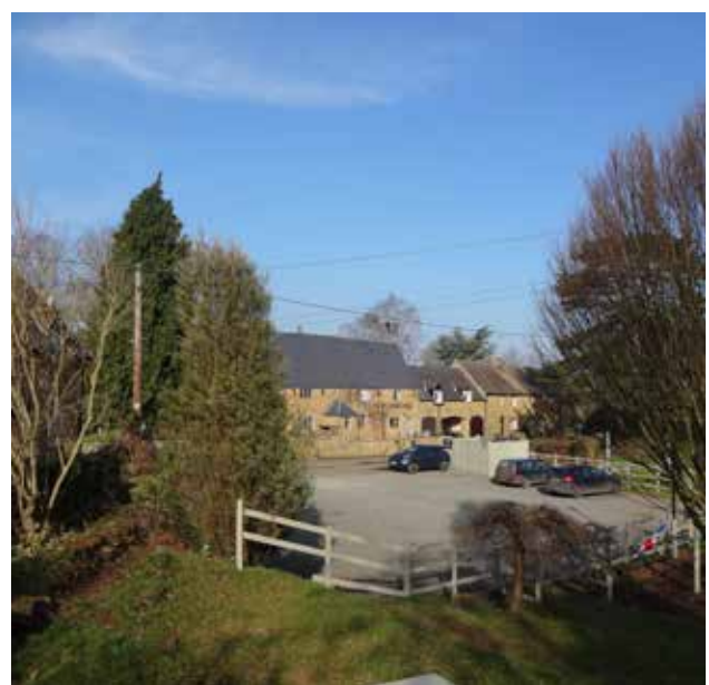
View from Milton Road across Inn Carpark
