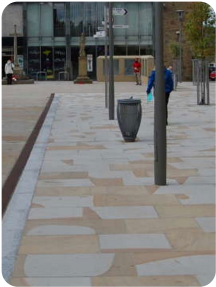
(01) Improved footways, using Yorkstone flag paving to match with style used in Sheep Street.
