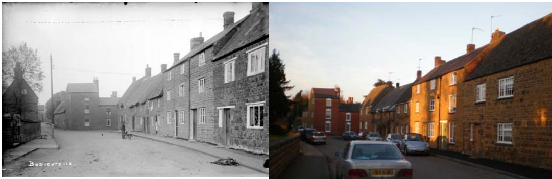
Looking north on Church Street
