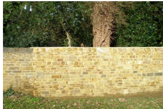
Wall to Bodicote House in Broad Gap
