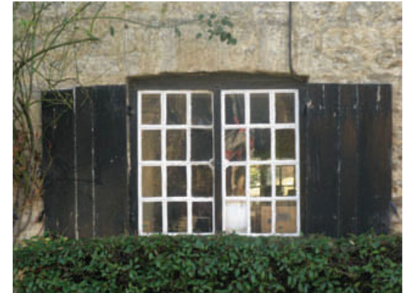
The windows of 3-6 Middle Street
