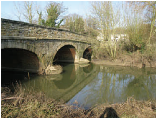
Islip Bridge from the southern bank
