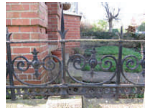
Railings on North Street
