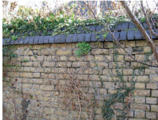
Blue bull nose brick used as coping
