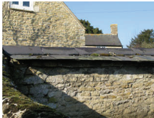
Large slates used as creasing/coping
