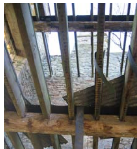
timbers inside Manor house ruins
