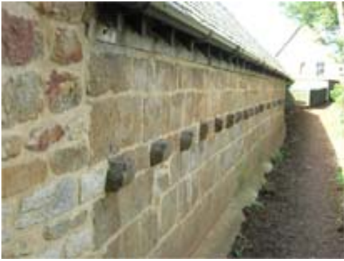
Church passage rustication
