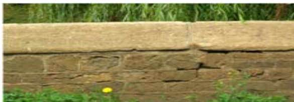
Old Bridge Road west enclosure wall
