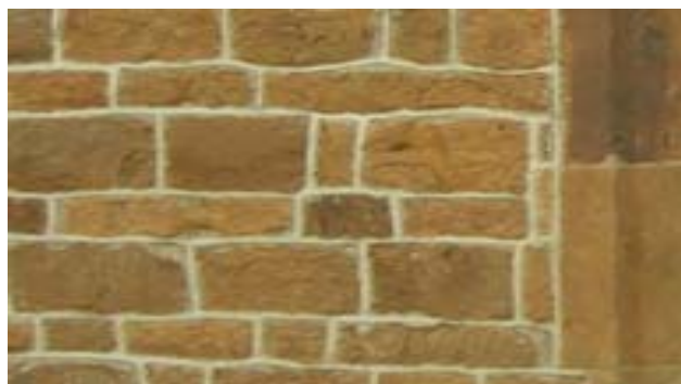
Above: bad pointing and the result; Below: an example of appropriate pointing
