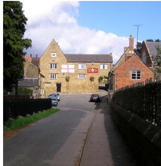
View north along Old Bridge Road
