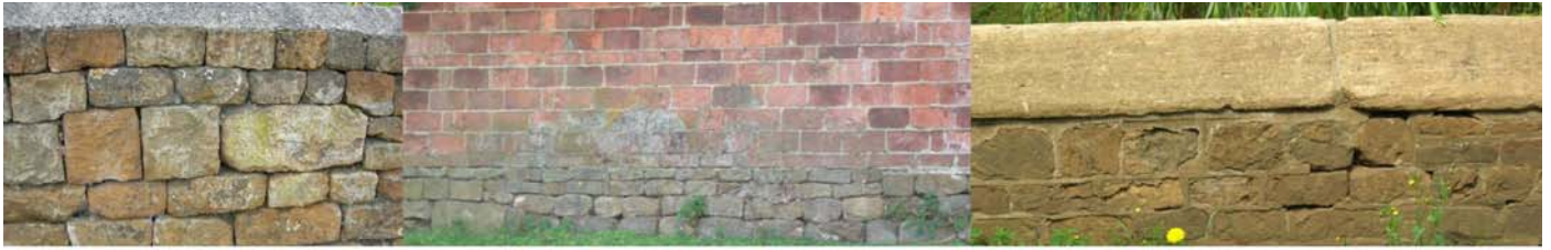
Marlstone wall, Cumberford road
