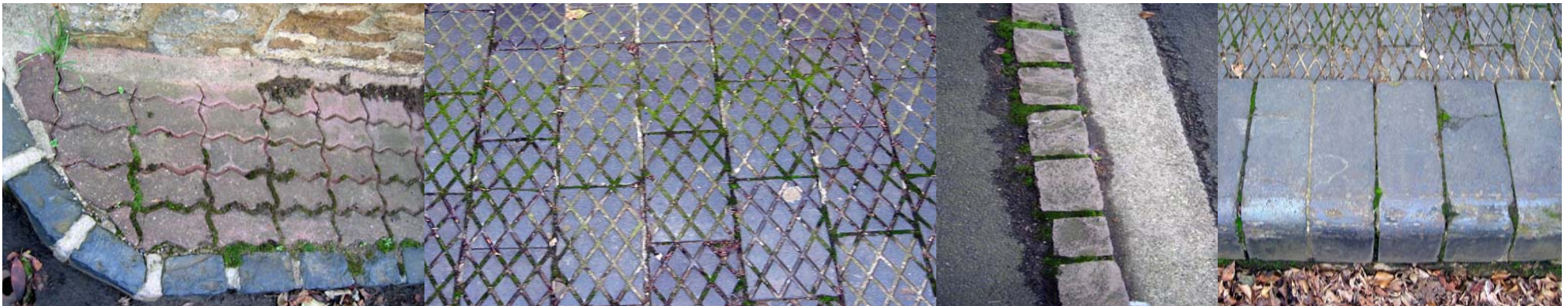
interlocking concrete paving with granite kerbs
