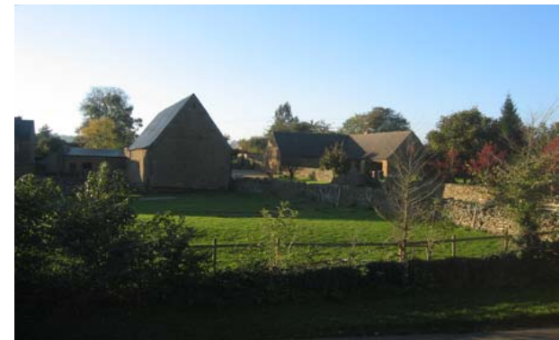
Scotland House from Claybank
