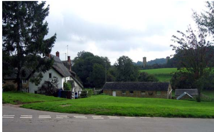
View to the south out of the conservation area.
