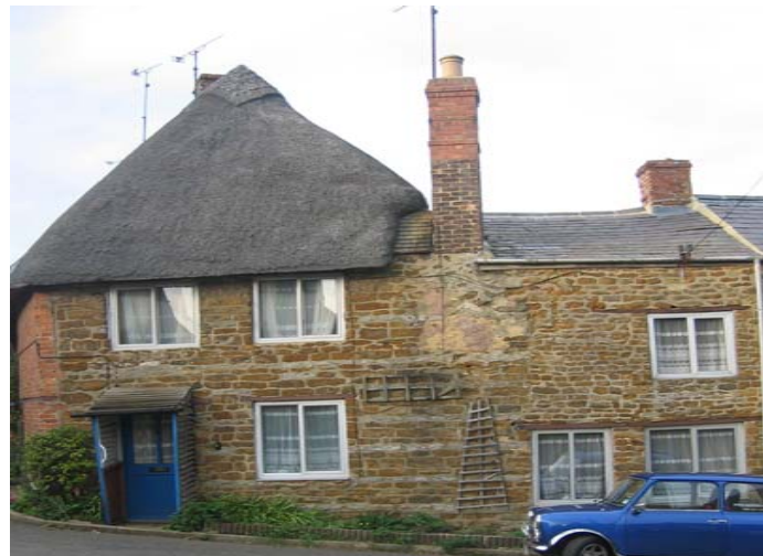
House on Down End showing a number of later additions
