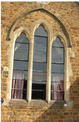
Window detail Old School
