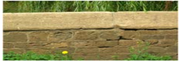
Old Bridge Road west enclosure wall
