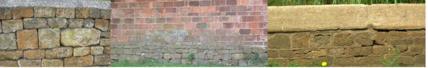
Marlstone wall, Cumberford road
