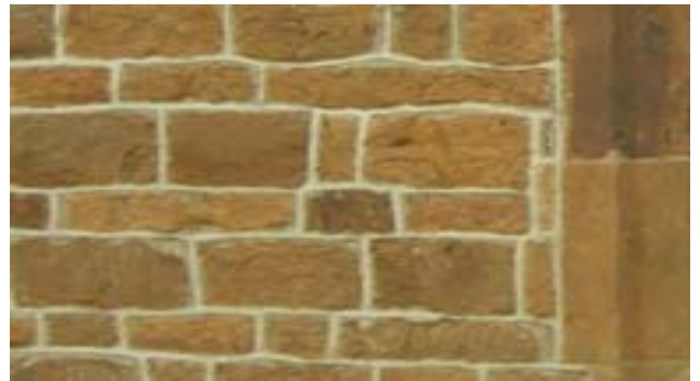
Above: bad pointing and the result; Below : an example of appropriate pointing
